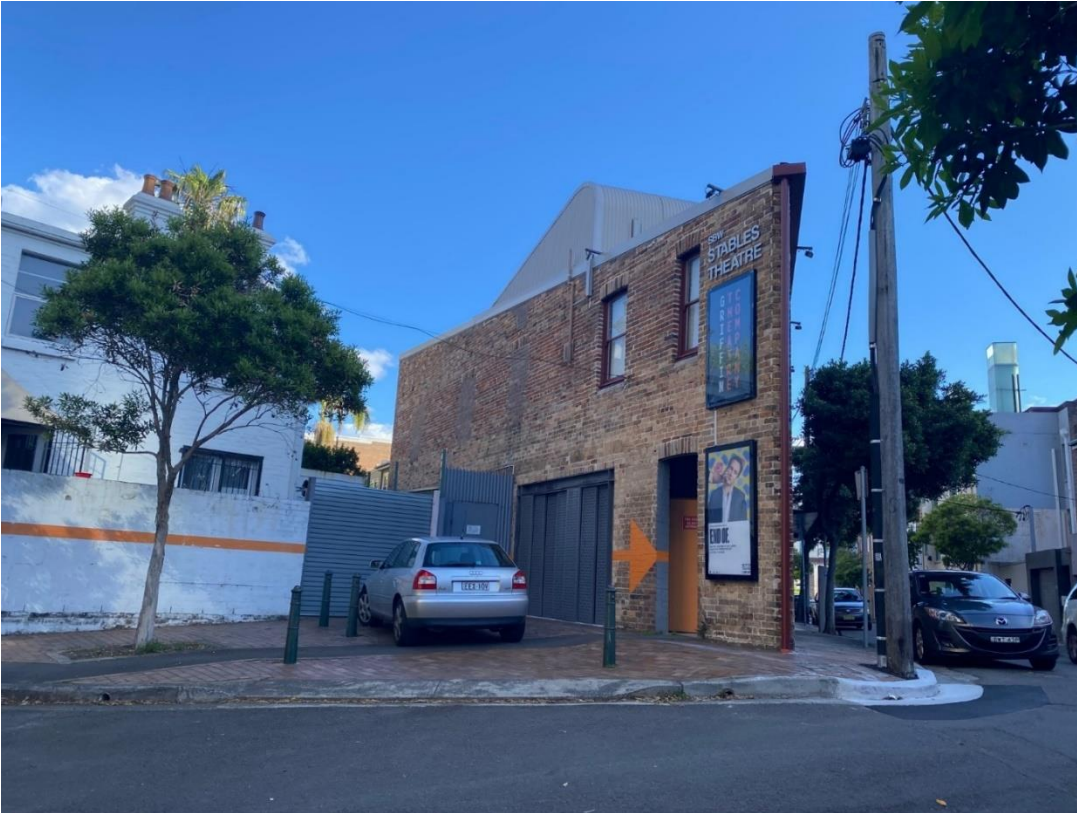
Figure 3. 10 Nimrod Street, viewed from the north-west
